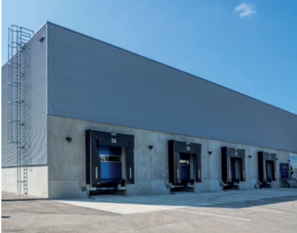
Truck loading bays at the ROTORCOMP LOGISTICS CENTER
